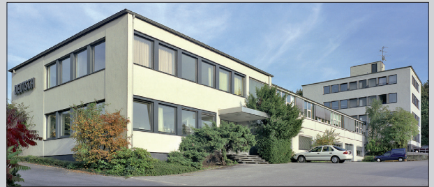
Works 1 (erected in 1967, extended in 1972) is the headquarter where the administration, the applications lab and electronics R&D are located. Portable test instruments, sensors and crack detection liquids are produced here.
