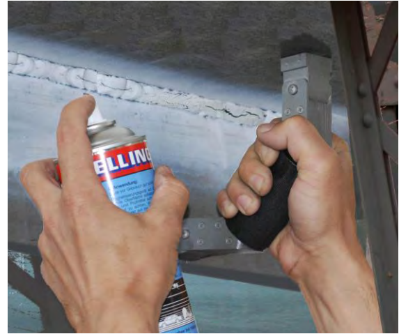
Weld joint inspection on a bridge by use of BW 333 black magnetic particle suspension and NR 104 A white background paint.
